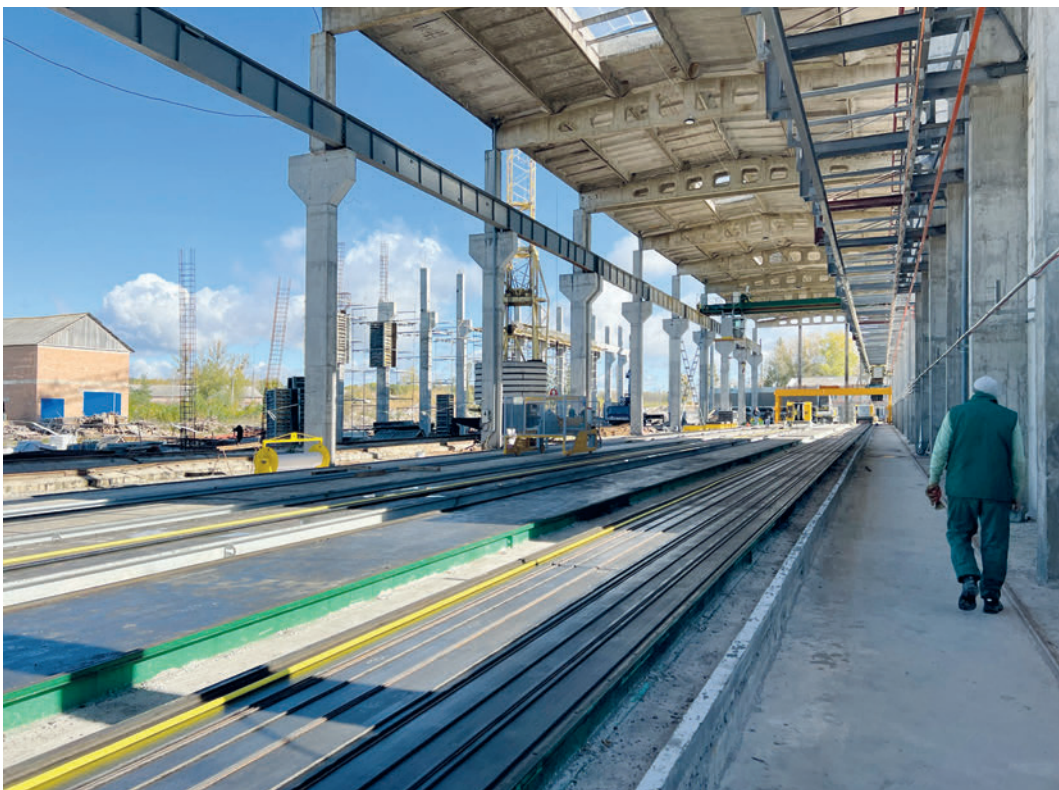
Hollow core slabs production line
