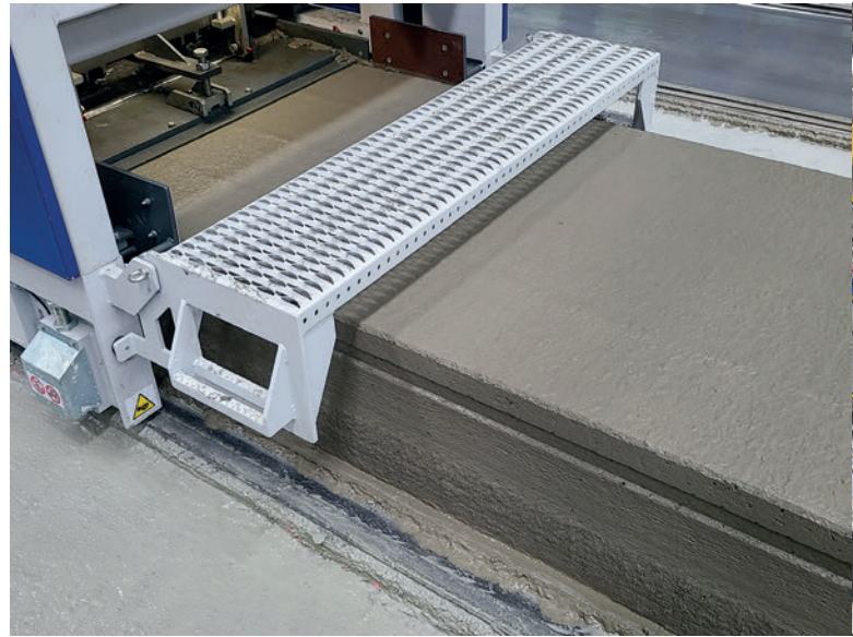
Casting of 500mm high hollow core slabs
